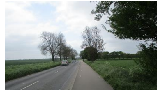
View of the existing route
